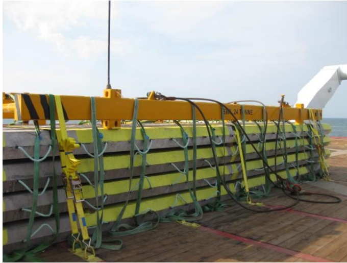
Figure 4 – Concrete mattresses and installation frame in stowed position on vessel
