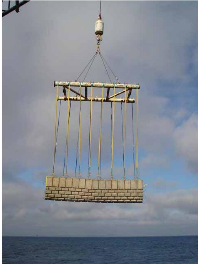
Figure 6 – Mattress and rigging arrangement prior to immersion in ideal installation conditions
