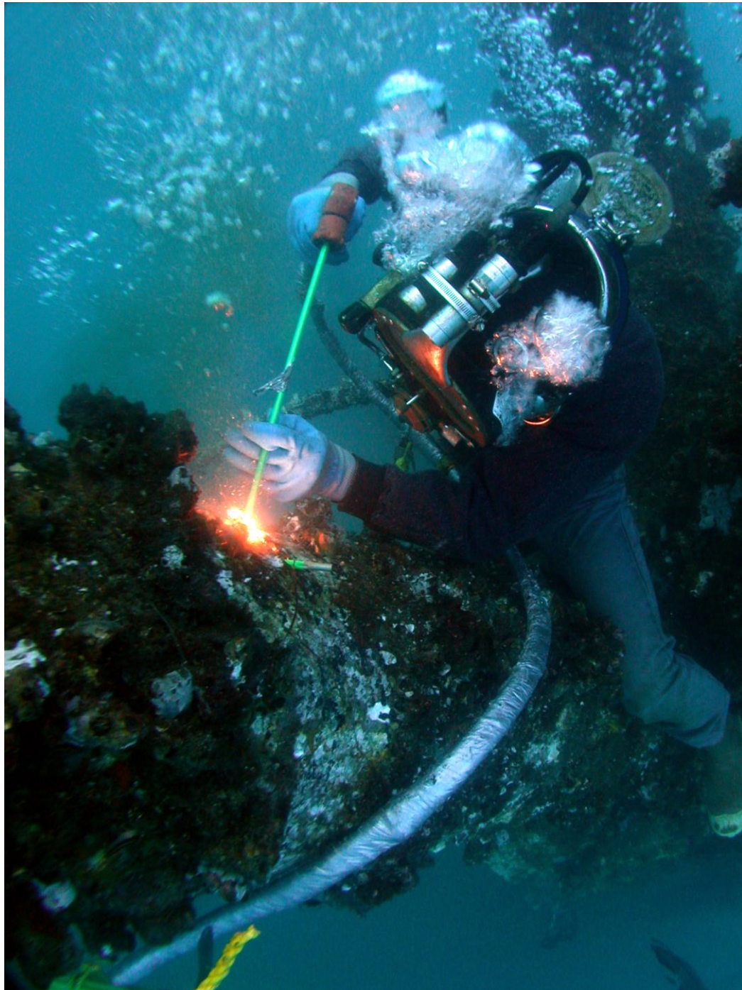
Diver using Oxylance AQUA EXO (Photograph reproduced with permission from Brian Derby: EPIC Divers)
